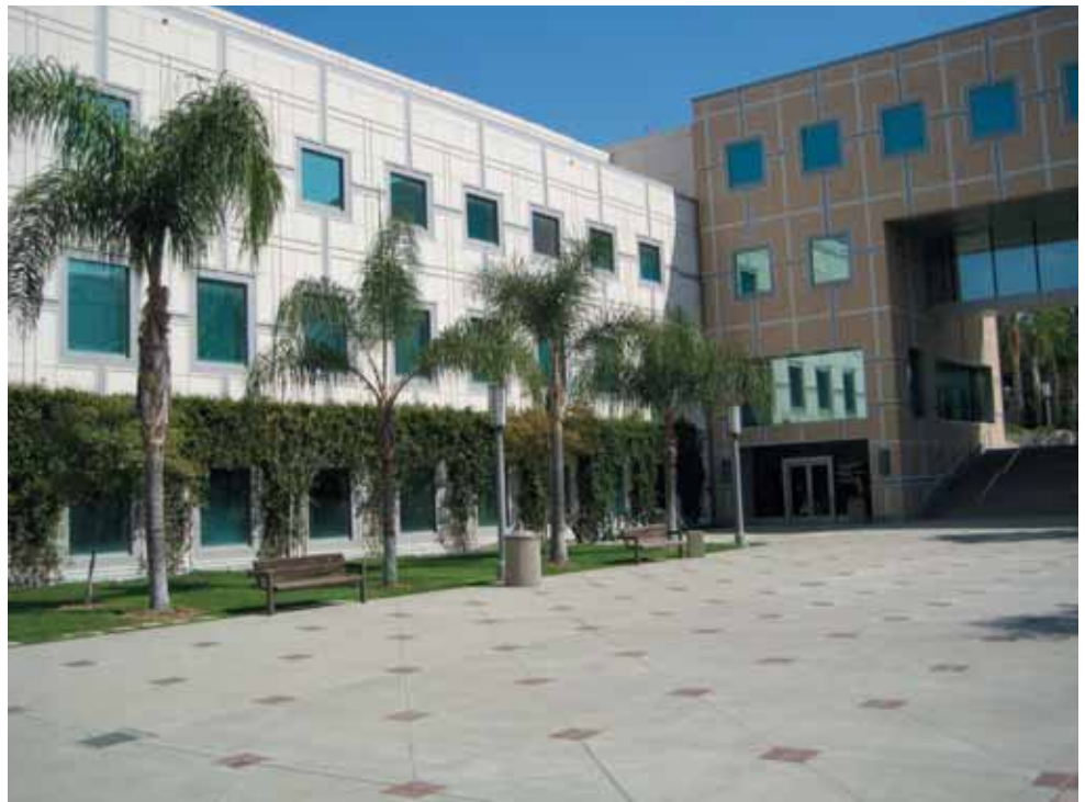
Department of Civil and Environmental Engineering
